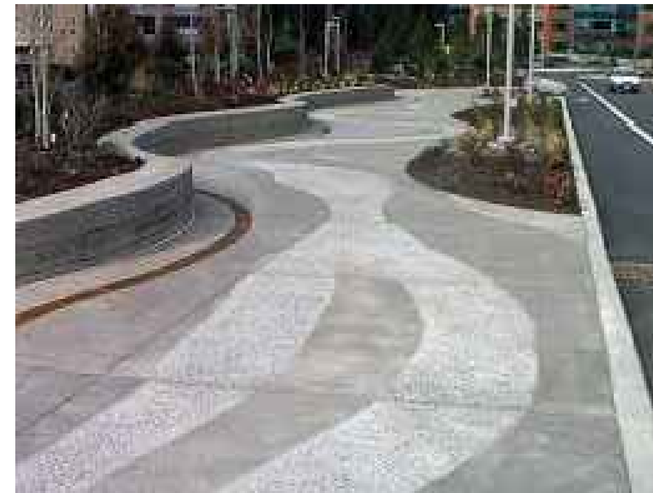
CONCRETE DRY STREAM PATH
