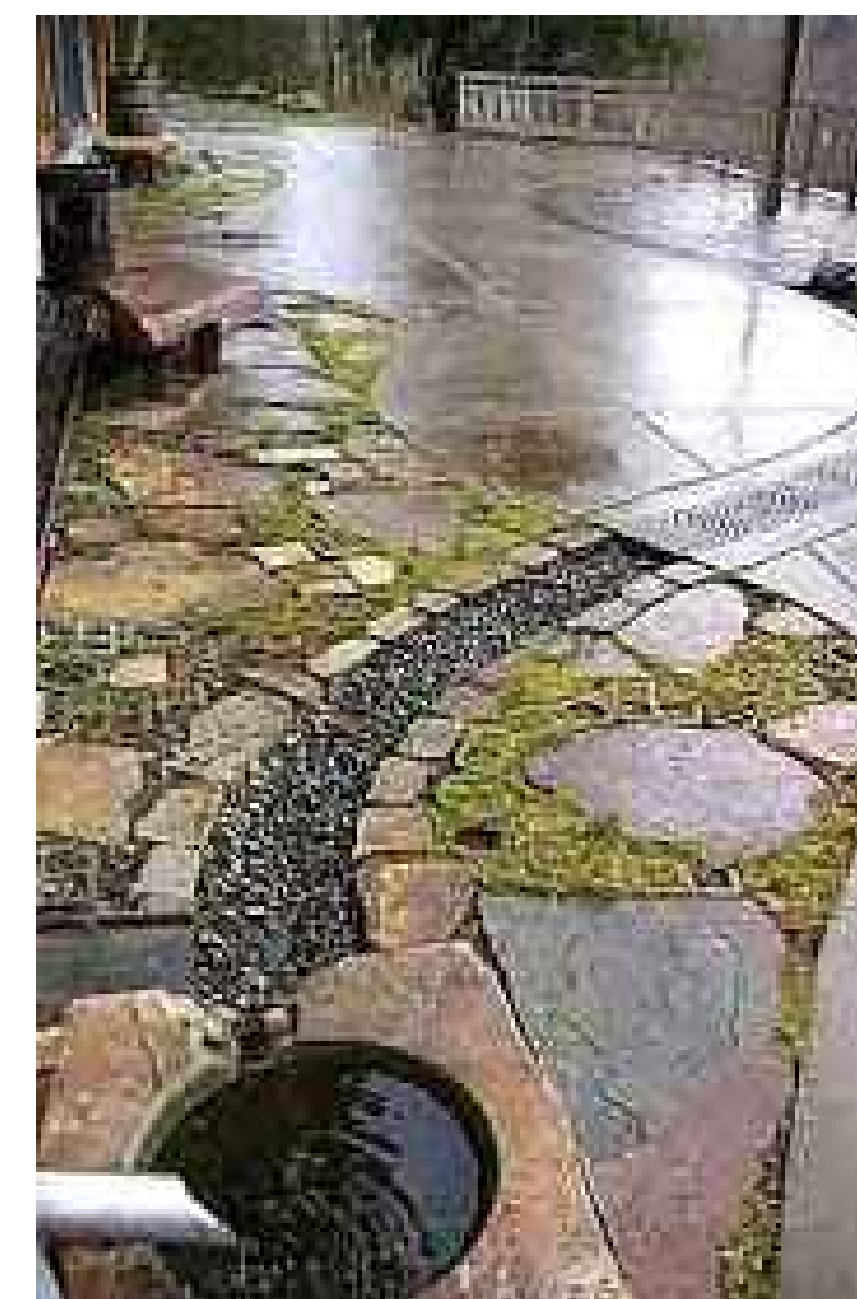
DOWNSPOUT RUNNEL
